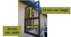
The net clear opening dimension requirements shall be obtained by the normal operation of the emergency escape and rescue opening from the inside, without special knowledge or tools.
