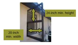
The net clear opening dimension requirements shall be obtained by the normal operation of the emergency escape and rescue opening from the inside, without special knowledge or tools.
