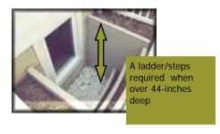
Bars, grilles, covers, screens or similar devices are permitted to be placed over emergency escape and rescue openings, provided such devices shall be releasable or removable from the inside without the use if a key, tool, special knowledge or force greater than that which is required for normal operation.
