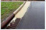
Inlet protection BMPs capture sediment before it enters the storm sewer.
