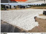
**Best Management Practices not maintained**  Unmaintained BMPs do not function properly and allow sediment to escape and enter waters of the state.
