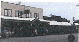
West side of Glover St - diagonal parking
